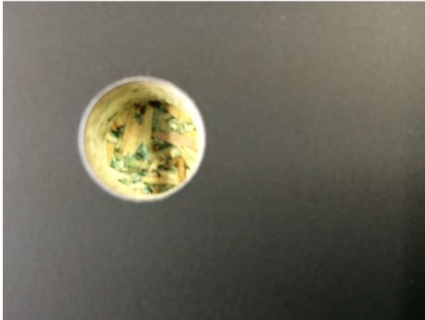
Blinde boring, diameter 16 mm
